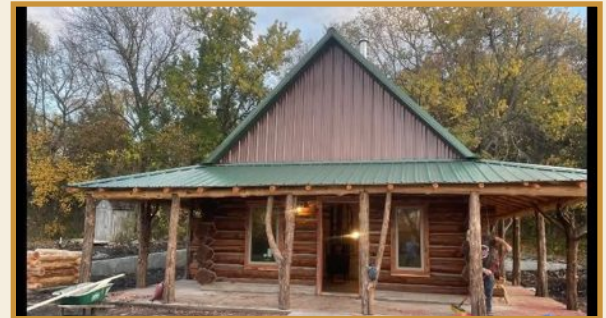
Completed cabins in the Camper's style
