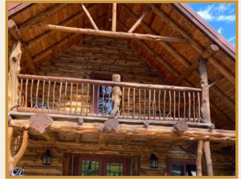
Exposed log trusses & gables
