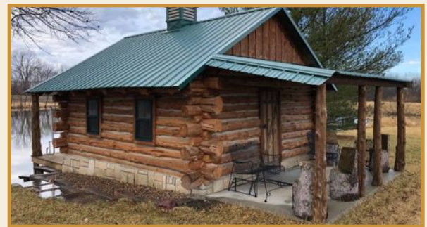
Full-log walls, metal roof, real notched corners
