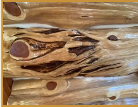
Hand-notched corners, flared butts
